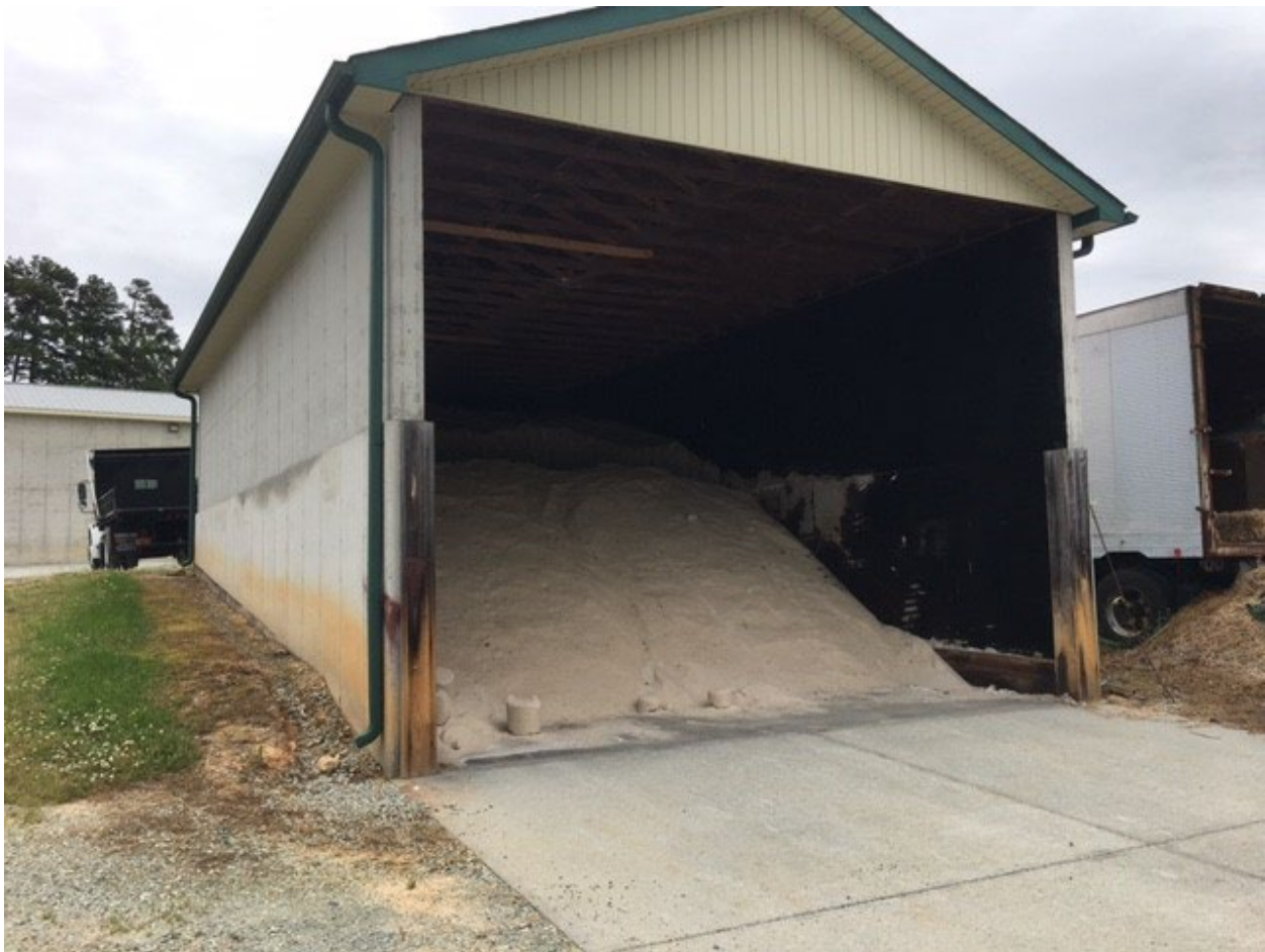
Salt Storage at Public Works
